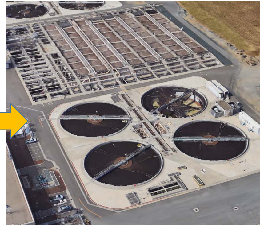
Treatment Plant for treatment and disinfection
