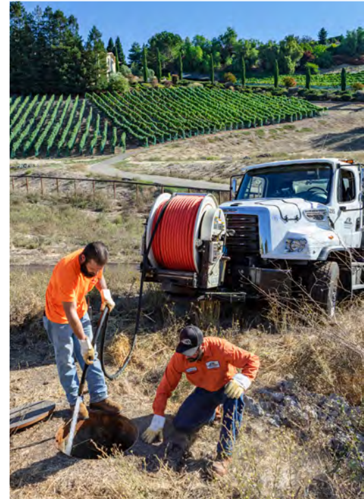
UPSTREAM: The Central San team releases the wipes into the sewer main.
