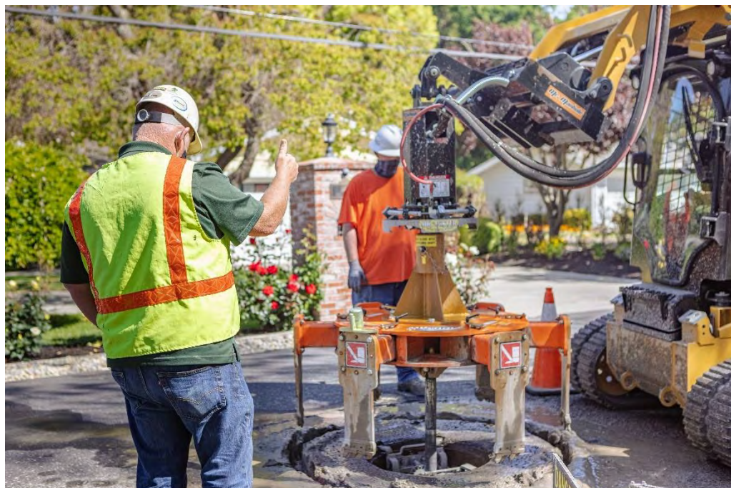
Figure 4.13: – Field Crews Resetting Structure Structure Height
