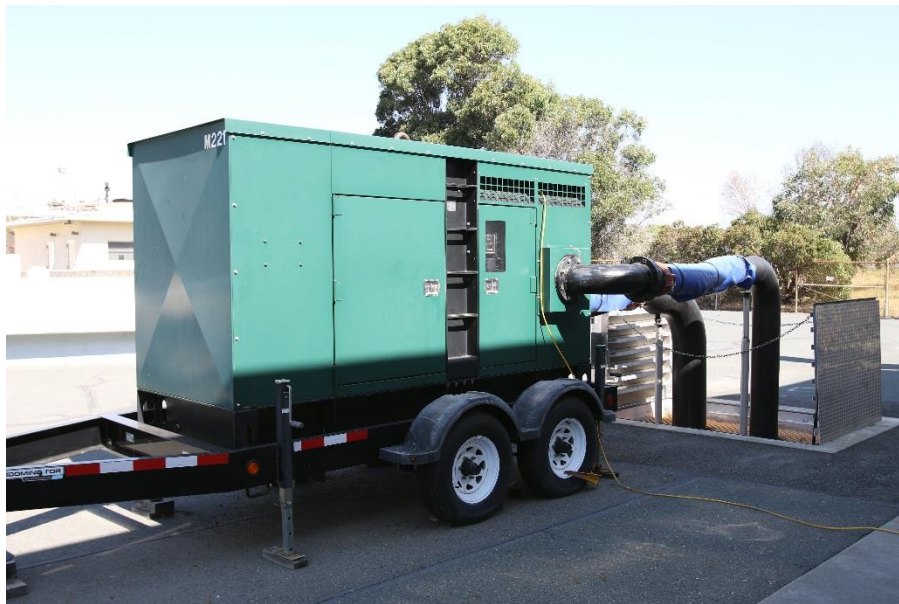
Figure 4.25: Portable Emergency Bypass Pump at Martinez Pumping Station
