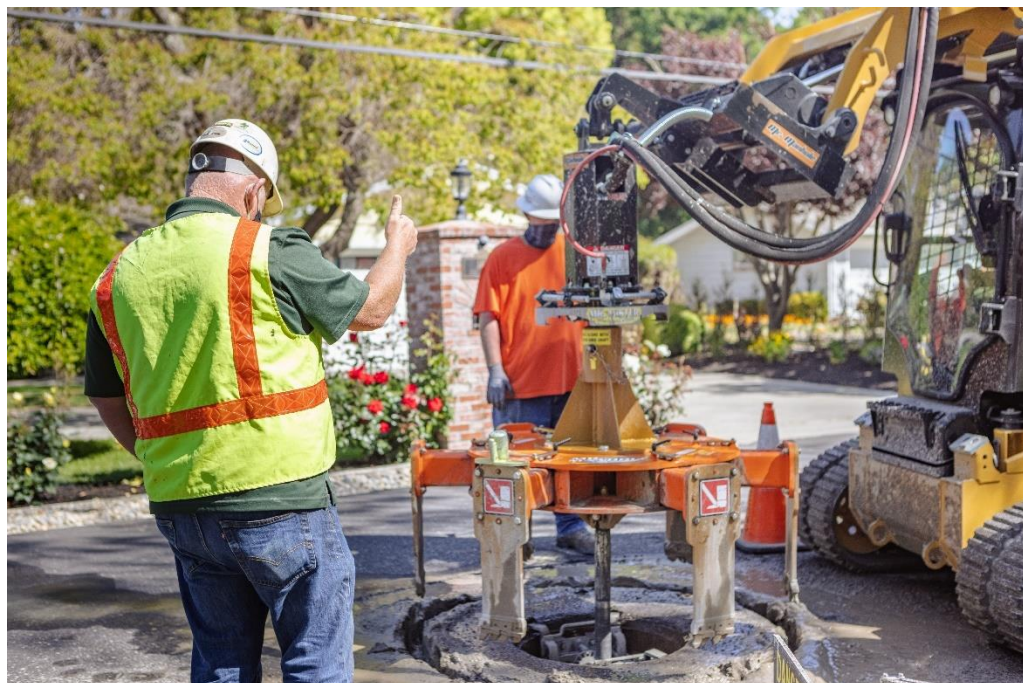
Figure 4.13: – Field Crews Resetting Structure Structure Height
