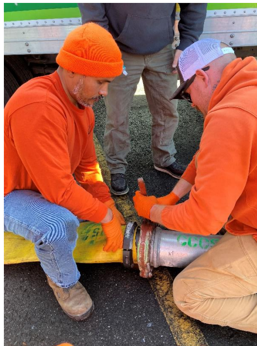
Figure 4.18: Victaulic Pipe Coupling Training Exercise
