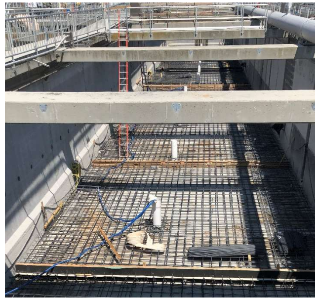
Construction progress for the new aeration diffusers and seismic improvements under the Aeration Basin Diffuser Replacement – Phase 1, District Project No. 100019.
