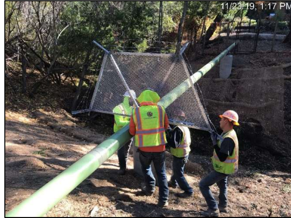
Sewer Replacement in a Residential Neighborhood and Aerial Creek Crossing
