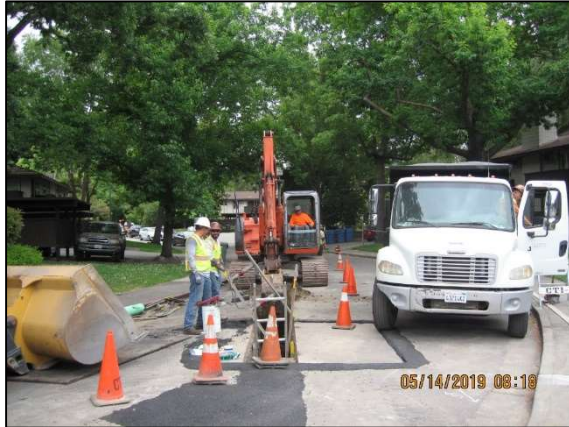
Sewer Replacement in a Residential Neighborhood and Aerial Creek Crossing
