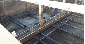
corroded reinforcing bars, and show signs of significant cracking. Some concrete areas require coating to prevent further corrosion. This project is to address these aging infrastructure needs and improve the safety and reliability of existing systems.
