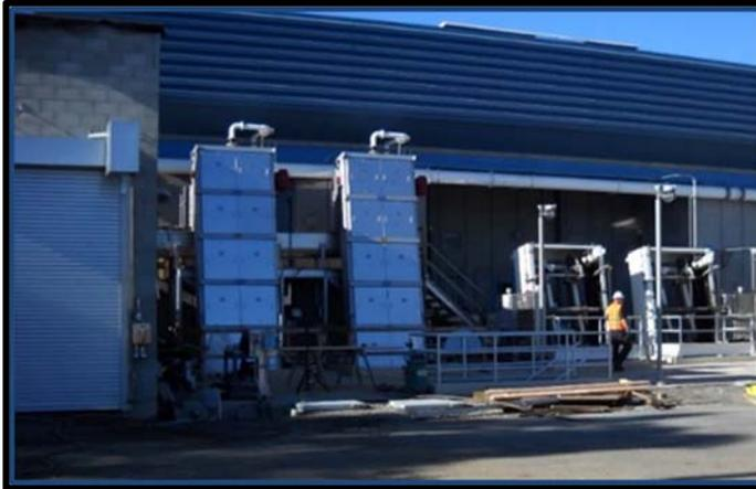
*New Screens Installed for the Headworks Screening Upgrades Project*
