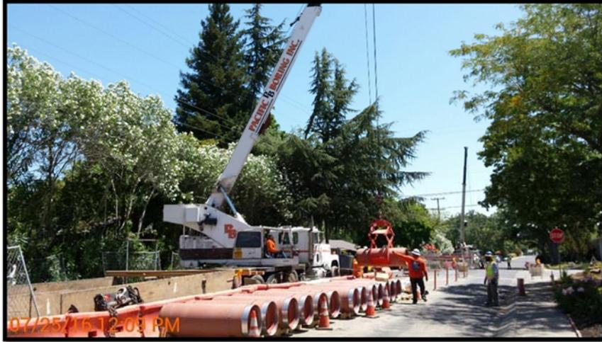
*Sewer Installation in Pleasant Hill Using Pilot-Tube Boring*
