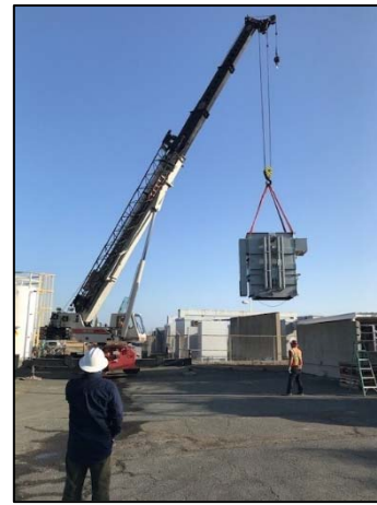
Constructing new steel storage tanks and replacing a failed transformer under the Filter Plant and Clearwell Improvements Project – Phase 1
